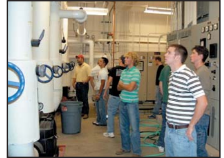
Students view the mechanical systems at the Henry Doorly Zoo's heating and chilling plant.
